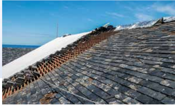
CAMPS BAY HIGH SCHOOL ROOF REPLACEMENT 2016
